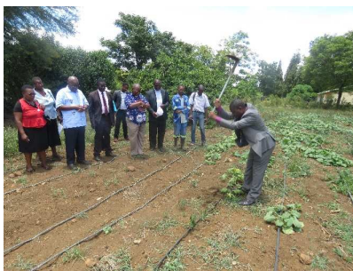
The Rt. I. Mukuwanda Ground Break for 1000sqm green house project at Habern park
